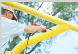
Level then Drill and Bolt "T" Adapter In Place
