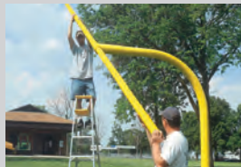
Tip Crossbar to Level and Clamp
